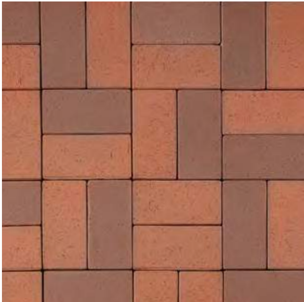
Blockverband (2er-Block)
